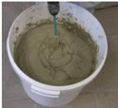
Mix the mortar with an agitator. Put comp. A + B into a 30l pail and mix thoroughly for 2 minutes- done.
